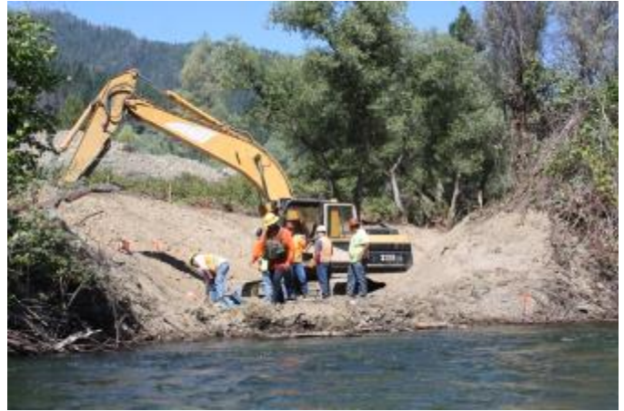
Restoration construction on the Trinity River. Photo © Ian Ausprey
